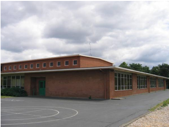
North and east elevations showing gymnasium
