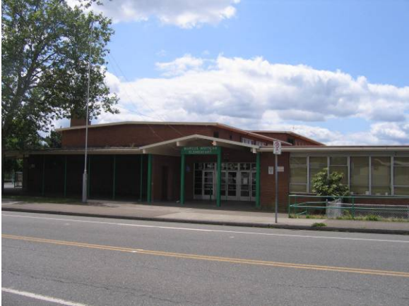
East elevation facing west
