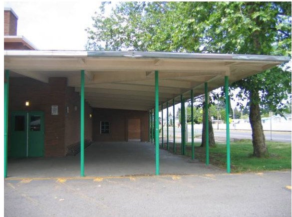
North elevation facing southeast
